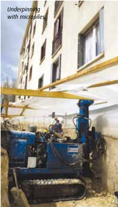
Underpinning with Fondopieu
