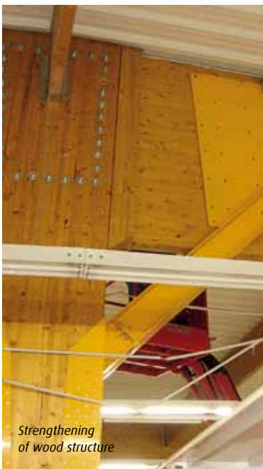
Floor strengthening with Foreva®TFC
