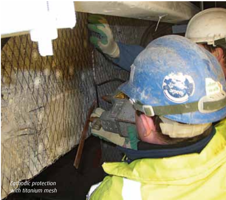
Waterproof repair in a cement plant
