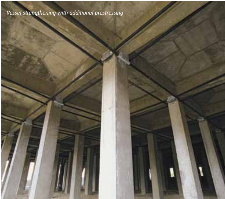
Water tower strengthening with additional prestressing loops
