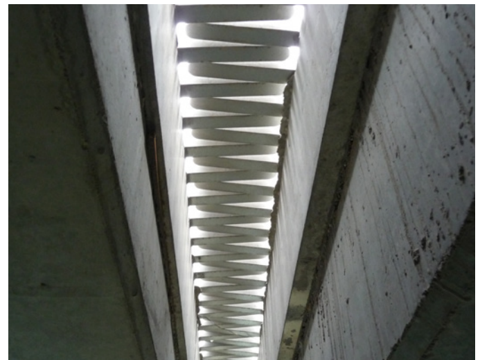
WP joint seen from below
