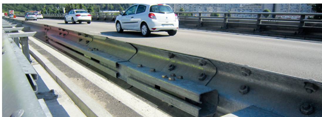
Application on a guardrail
