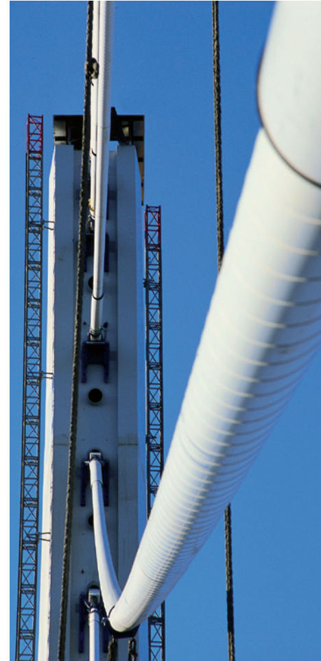
Helical fillet Millau bridge / France
