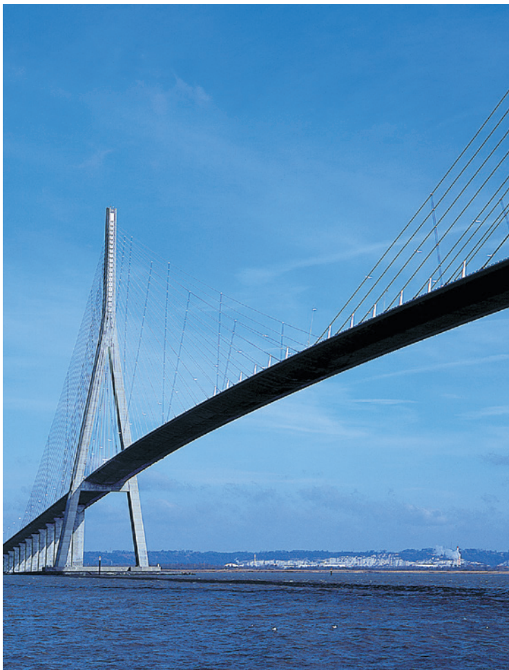
Normandie bridge cross tie / France
