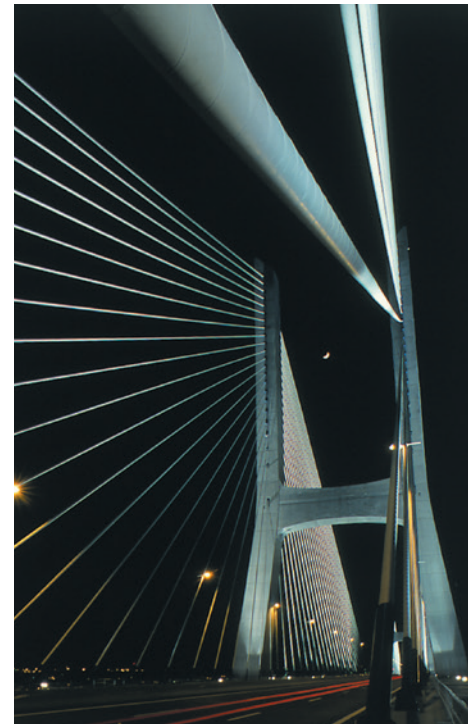
Light fittings Vasco de Gama bridge / Portugal
