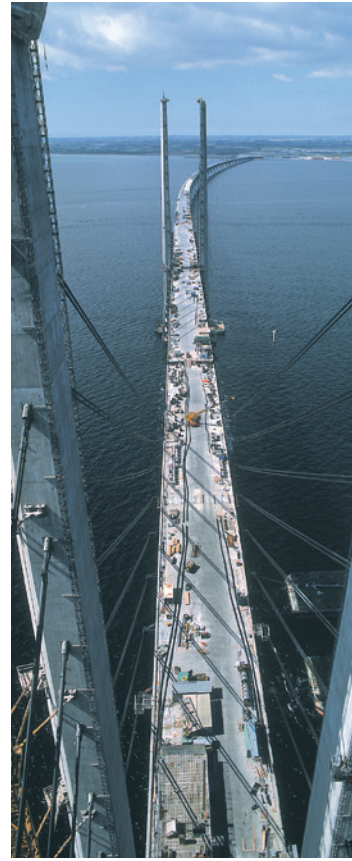
Øresund bridge Denmark-Sweden
