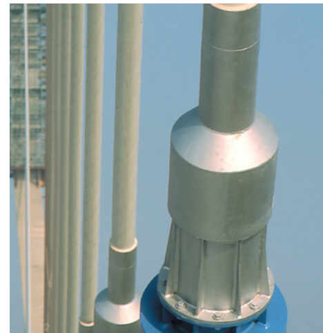
Antivandalism tubes Seohae Grand bridge / South Korea
