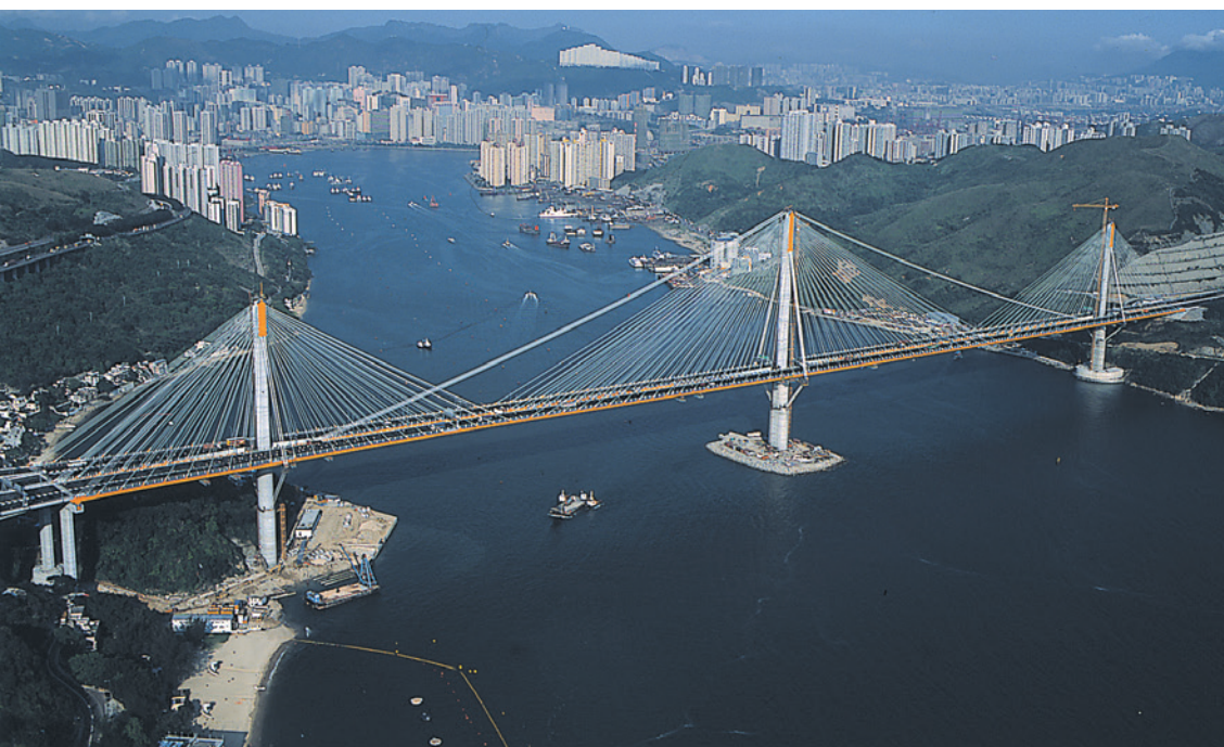
Ting Kau bridge / Hong Kong
