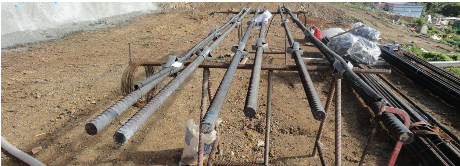
Preparation of Freyssi500 soil nails - Martinique, France
