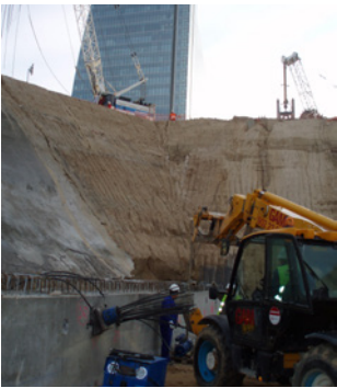
Tensioning strand anchors - International Convention Centre, Madrid - Spain
