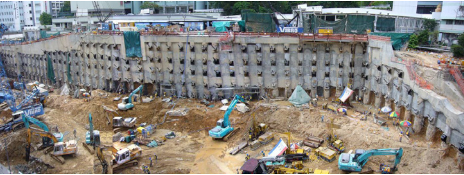
SBMA removable strand anchors - Phase II refurbishment of the Caritas Medical Centre - Hong Kong
