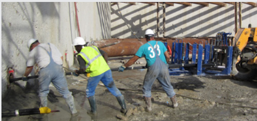
Strand anchor uncoiler
