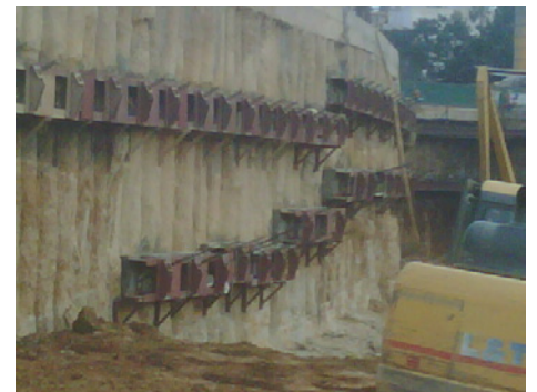
Temporary strand anchors - Bangalore Metro - India
