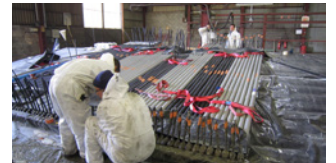
Production of permanent Freyssibar anchors
