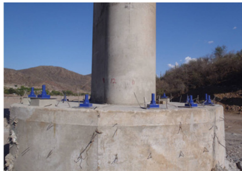
Self-drilling anchors, Batopilas Bridge - Mexico
