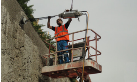
Tensioning of strand anchor, Rosa Parks OA9, Paris
