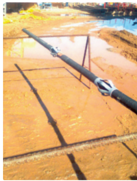
Preparation of a Freyssibar permanent anchor - Canadian Embassy, Rabat - Morocco
