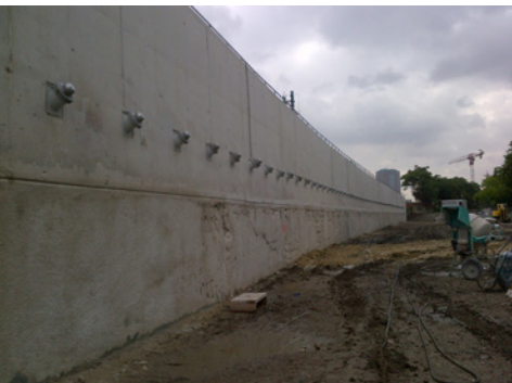
Permanent strand anchors - Rosa Parks station - France
