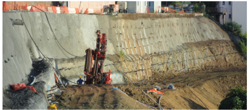
Freyssi500 soil nails - Morne Calebasse - France
