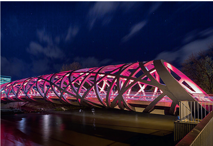
Hans Wilsdorf Bridge Geneva, Switzerland
