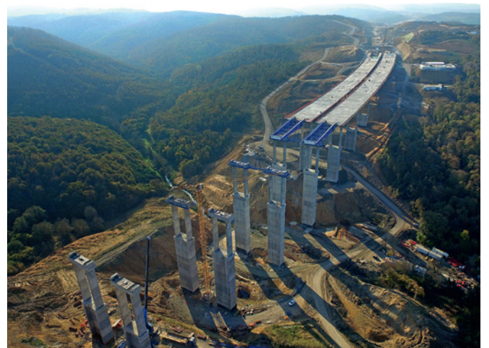
Third Istanbul Bypass Turkey
