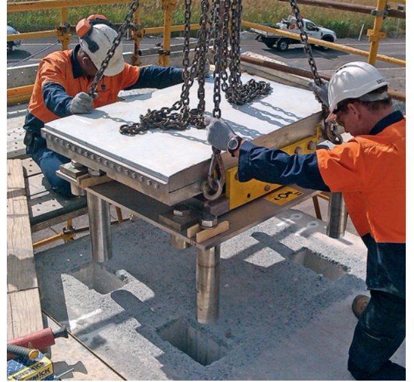
Gerringong Bridge Australia
