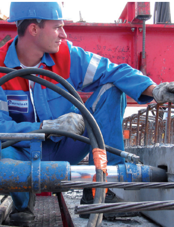
Sioule Viaduct, France
