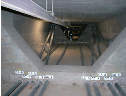
HDPE ducts for external prestressing
