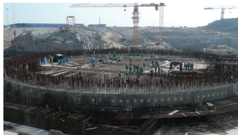
Nuclear containment vessel, China
