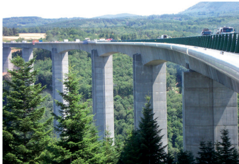
Sioule Viaduct, France
