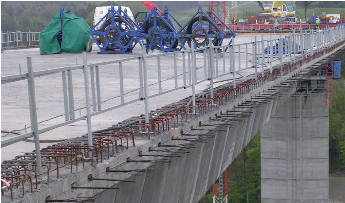
Bridge at Rousson, France
