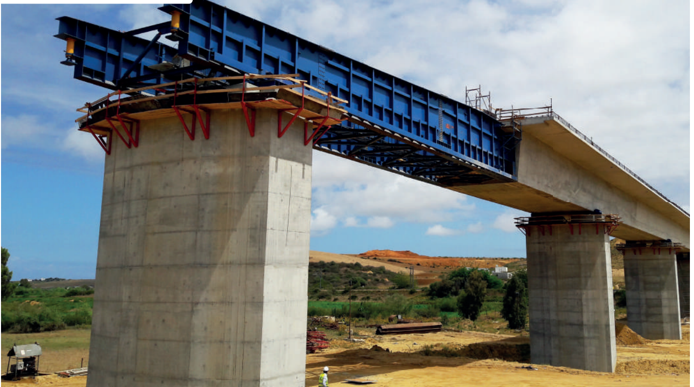
Tangier-Kenitra high-speed railway line, Lahlou viaduct Morocco
