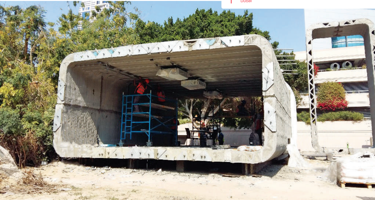
Office of the Future Prestressed assembly of 3D-printed elements Dubai
