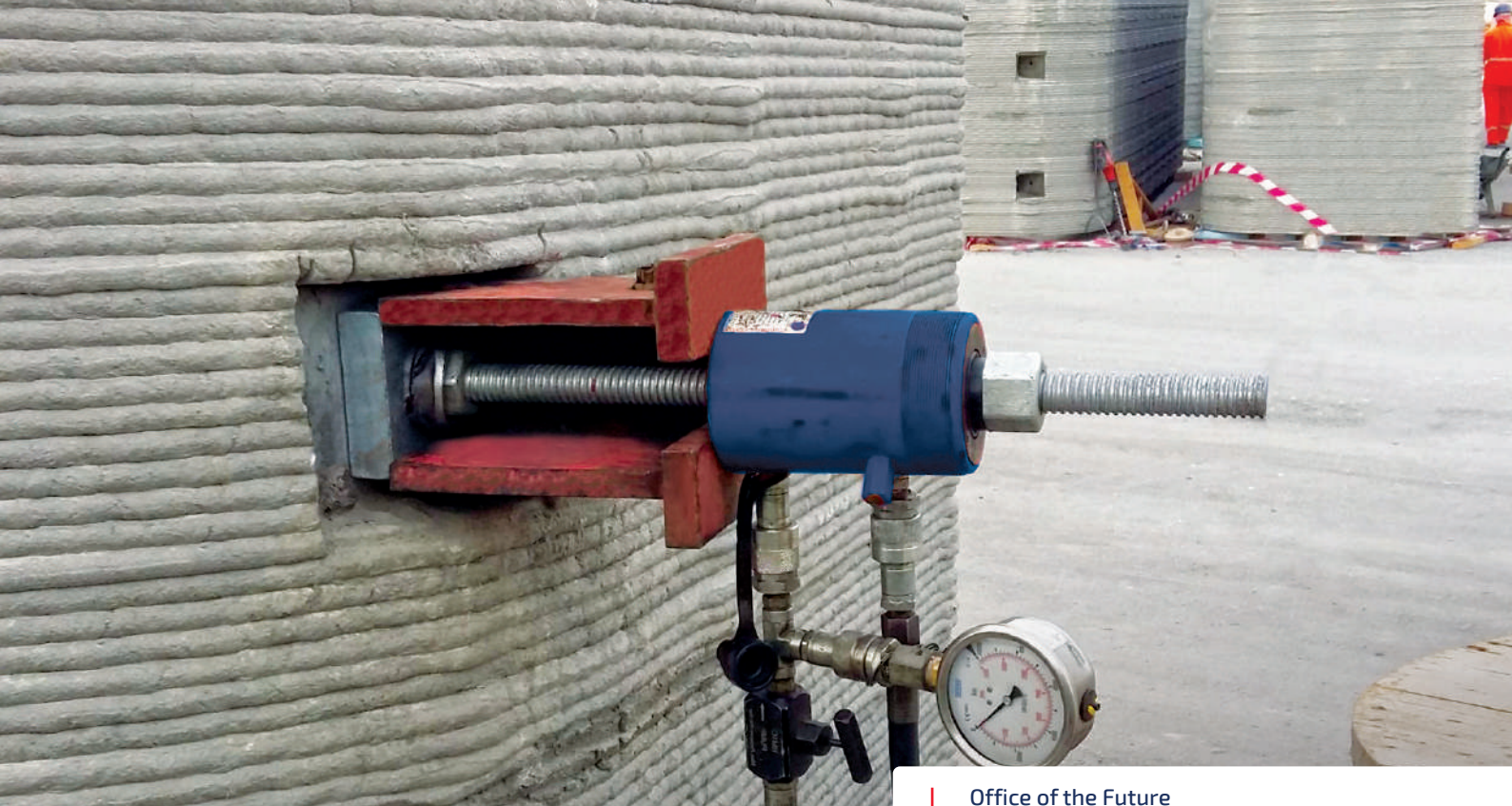
Office of the Future Prestressed assembly of 3D-printed elements Dubai
