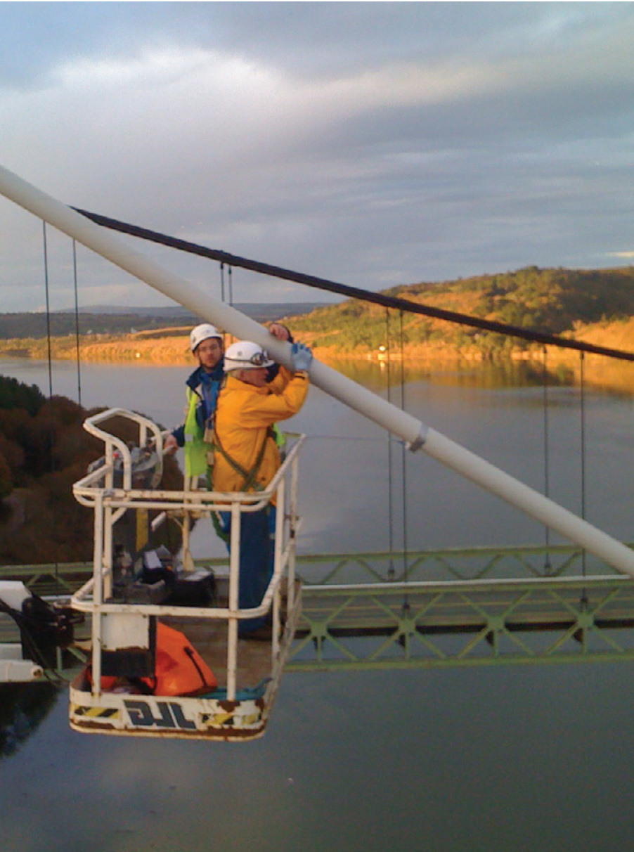
Visual inspection of stay cables
