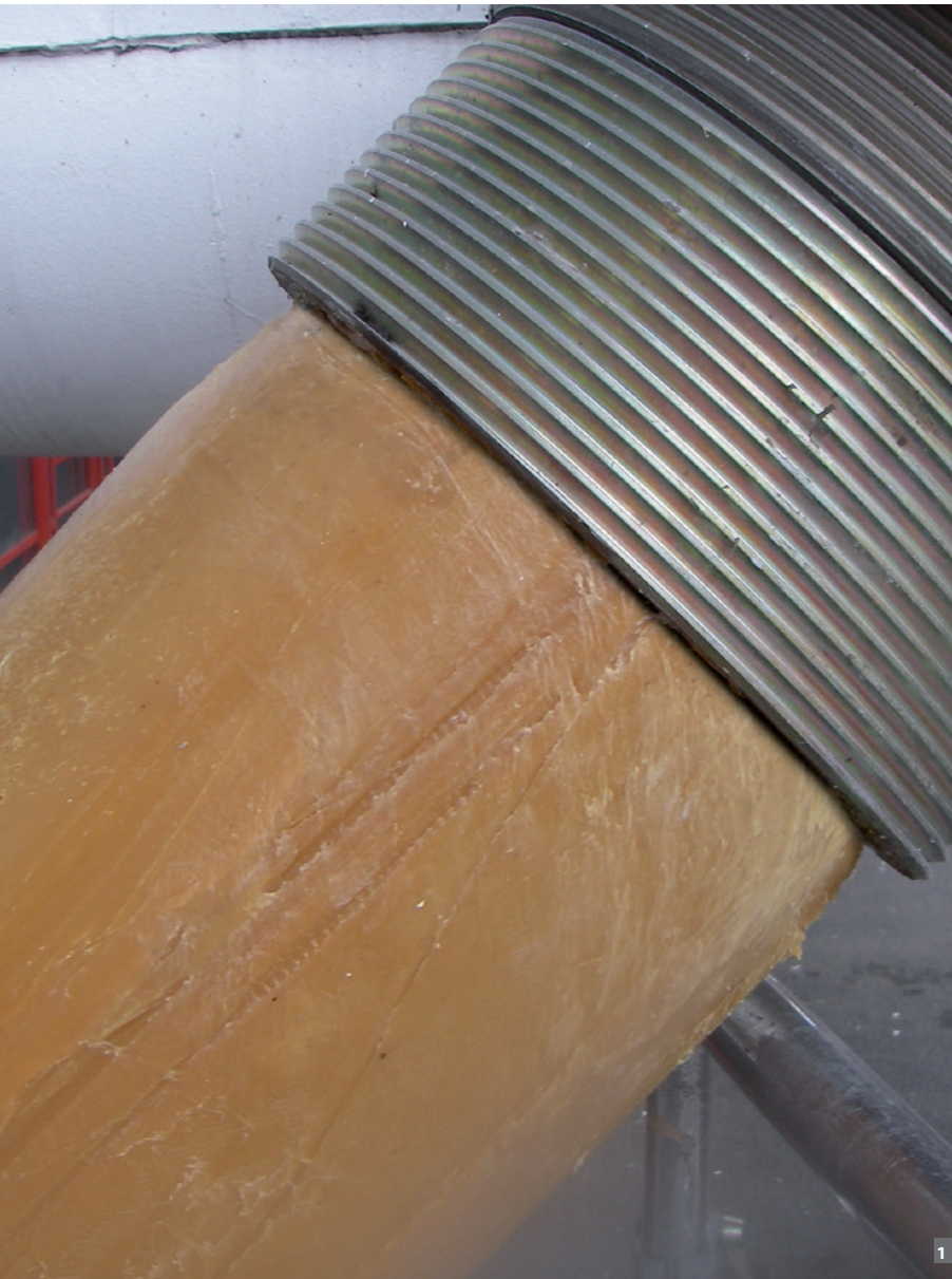
Opening of anchor covers for inspection
