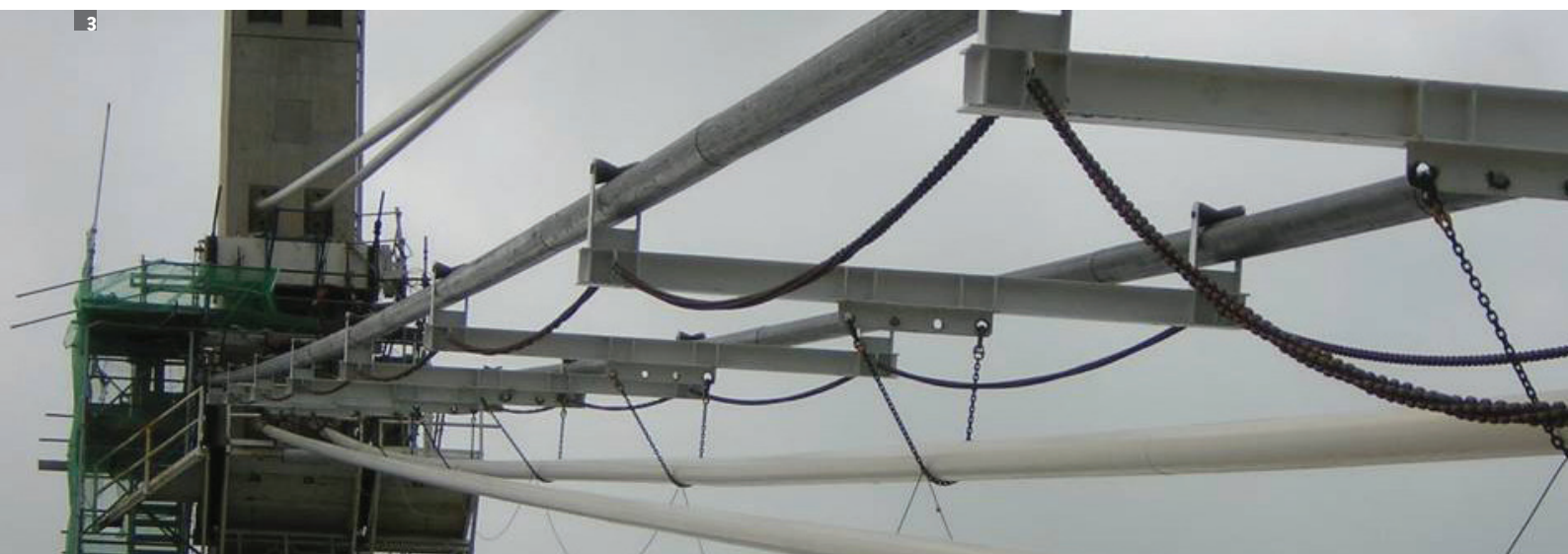
1 - Stay cables damaged by a vehicle fire 2 - Temporary replacement cable 3 - Device for lowering cable to be replaced
