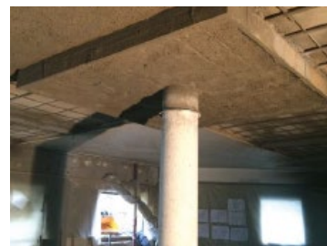
Office building, Noisy le Grand - FRANCE Underpinning of foundations | Shotcrete | TFC®
