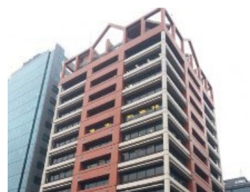
Customhouse Quay, Wellington - NEW ZEALAND Additional prestressing
