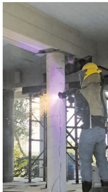
Simmon Apartment Building, North Carolina - UNITED STATES Corrosion protection
