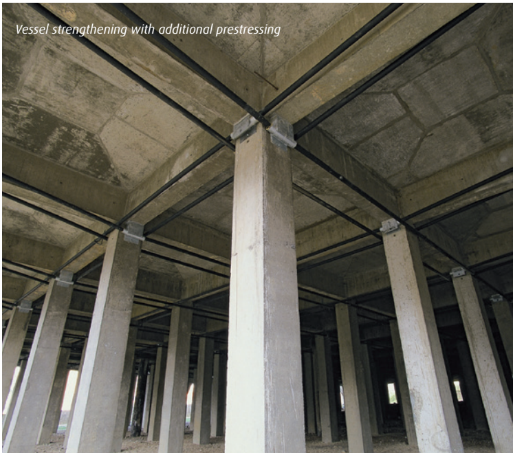
Water tower strengthening with additional prestressing loops
