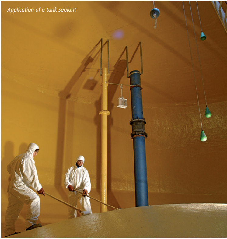
Strengthening metal tank for earthquakes with Foreva® TFC
